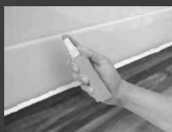
Mist the caulk bead and smoothing tool with SSK smoothing spray
